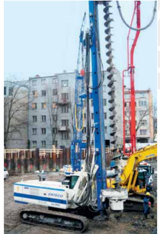
Tallin (ESTONIA) Centro commerciale E6050 – CFA240 Pali CFA ø 600-800 mm. Tallin (Estonia) New Shopping Mall E6050 – CFA240 rig model Drilled dia. 600-800 mm.
